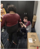
Easter Seals Office Work inside the Easter Seals office to build furniture.
