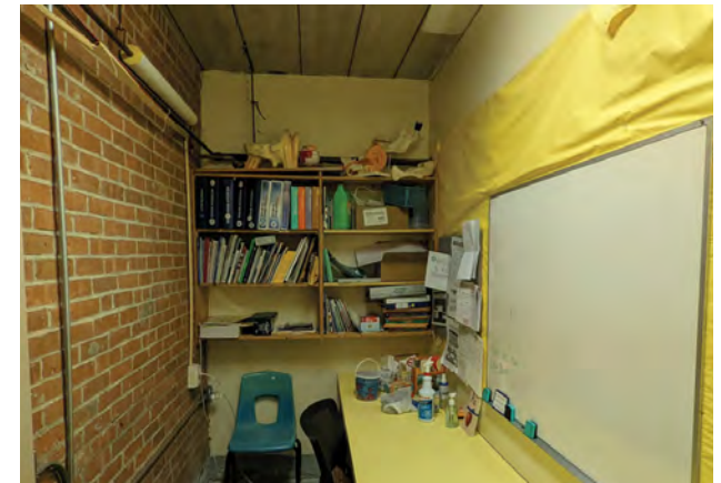
Undersized teacher work room located in basement (no elevator access)
