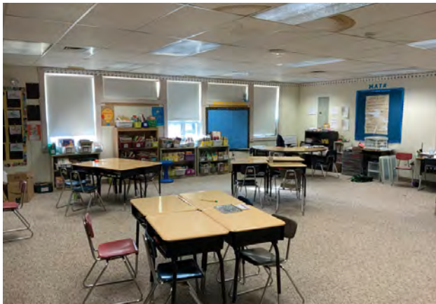
Modular classrooms house undersized kindergarten spaces with no toilet rooms
