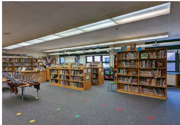
Former classroom re-purposed as media center; undersized
