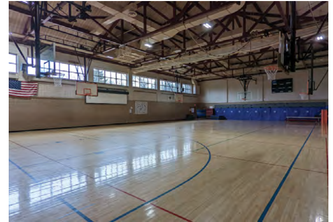
Gymnasium meets requirements, but associated storage and office spaces do not
