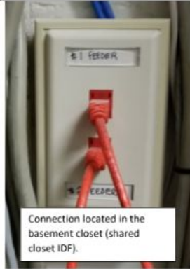
Network cables in basement IDF. Limited labeling.
